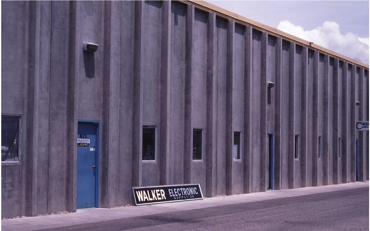
The temporary location at 3300 Princeton NE
