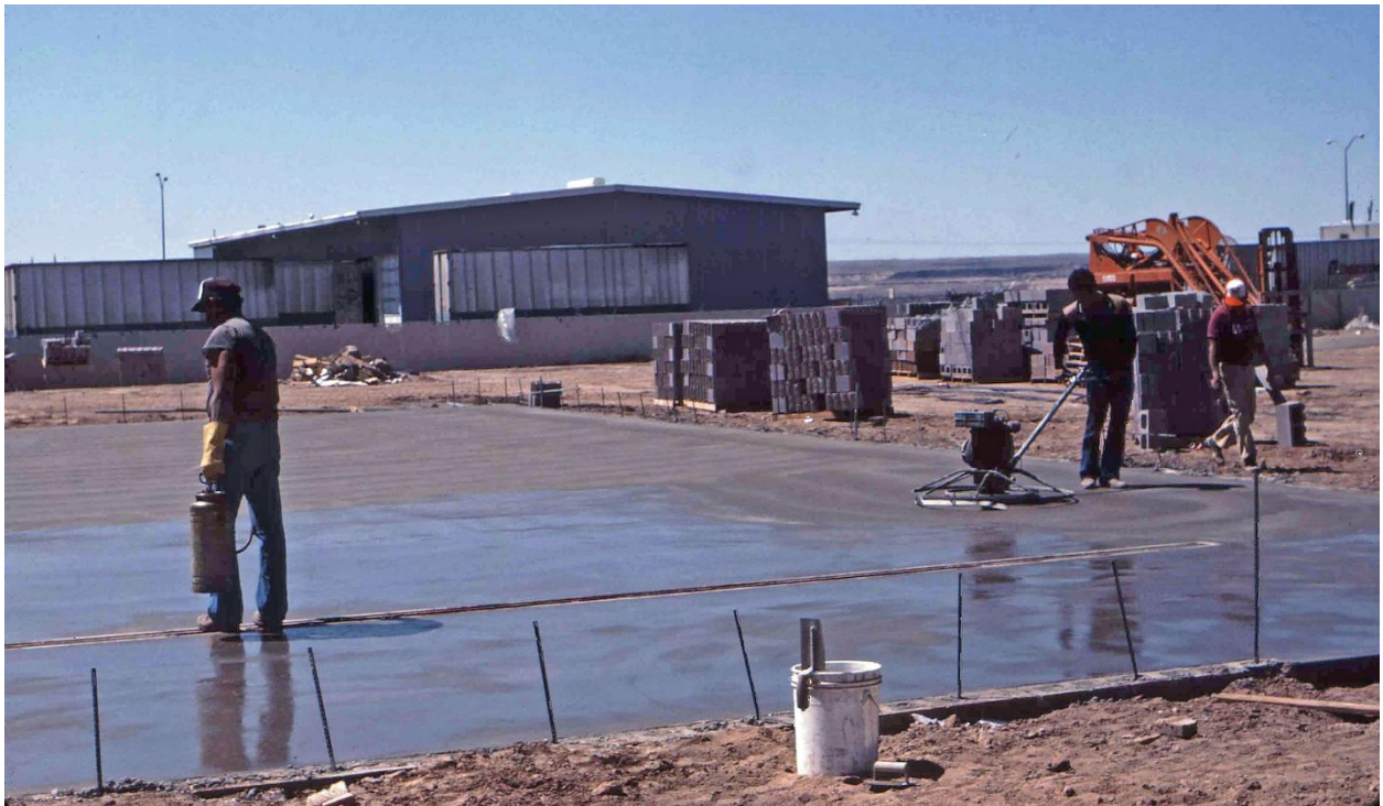
Beginning construction on the building at 3347 Columbia NE
