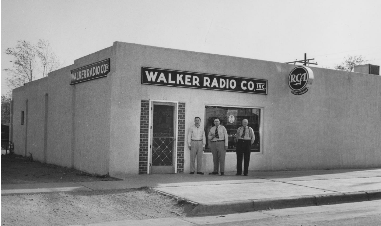
The building at 102 W. Granite, probably not long after Walker moved into it in 1954 John Hopperton,* Len Wilson, Bill Thomas
